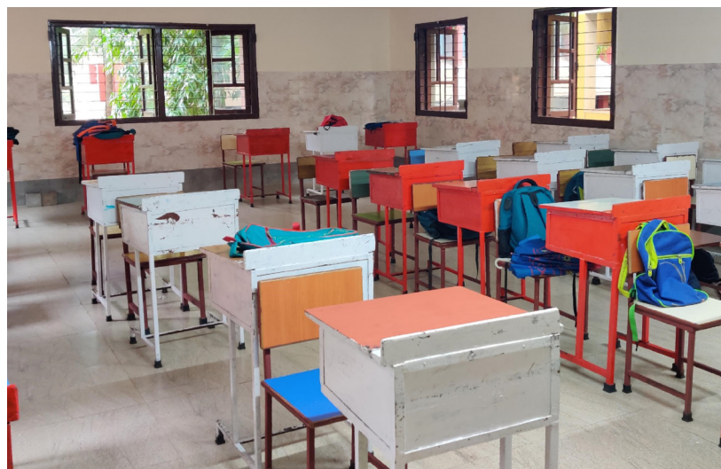
SDMS has contributed towards the refurbishment of toilets and study room at Agnells Balbhavan, Vashi, Navi Mumbai – a home for orphans and underprivileged boys through SHCIL Foundation.
